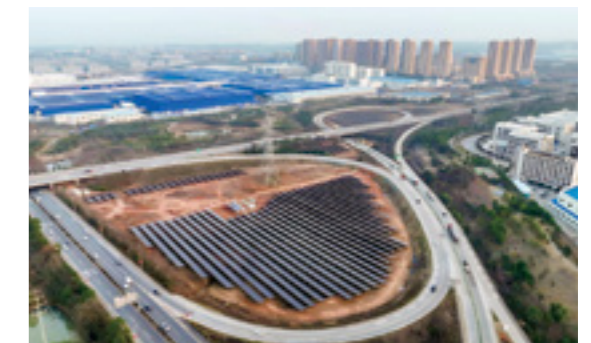
Distributed PV project at Huanghua Interchange of Hunan Changsha-Zhuzhou Expressway
