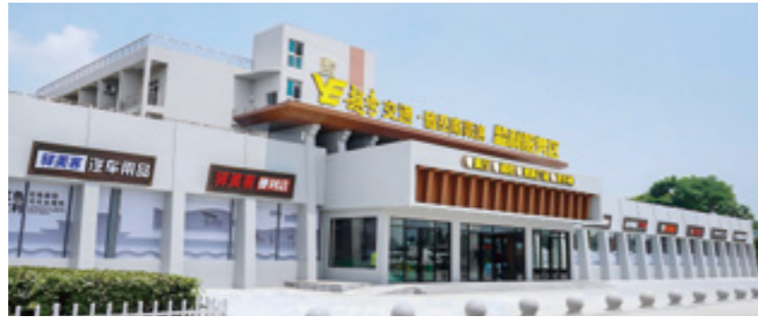
Upgraded Jianli Service Area
