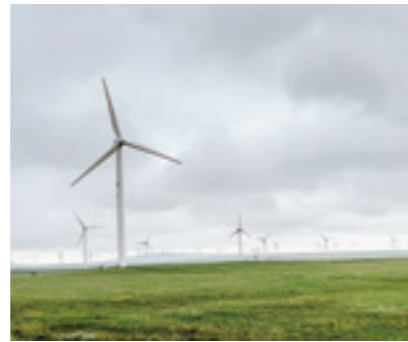
Yuexiu Financial Leasing wind power project
