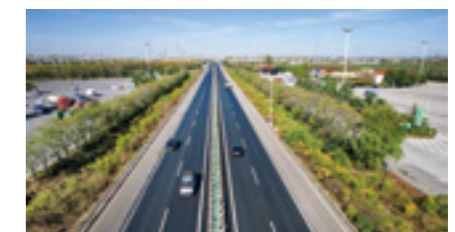
The deck of Shahe Grand Bridge after maintenance
