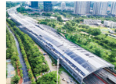
Guangzhou North 2nd Ring Expressway Full-Enclosure Noise Barrier Project
