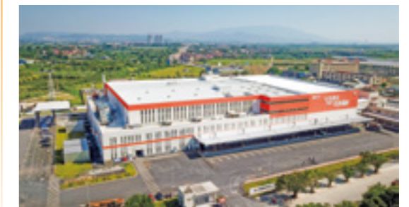
Fengxing Dairy Shitan Production, Research and Development Base
